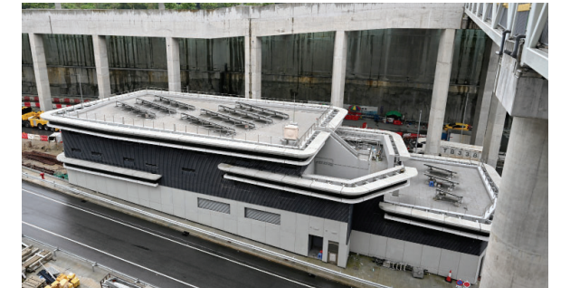
雨水泵房 Stormwater Pumping Station
