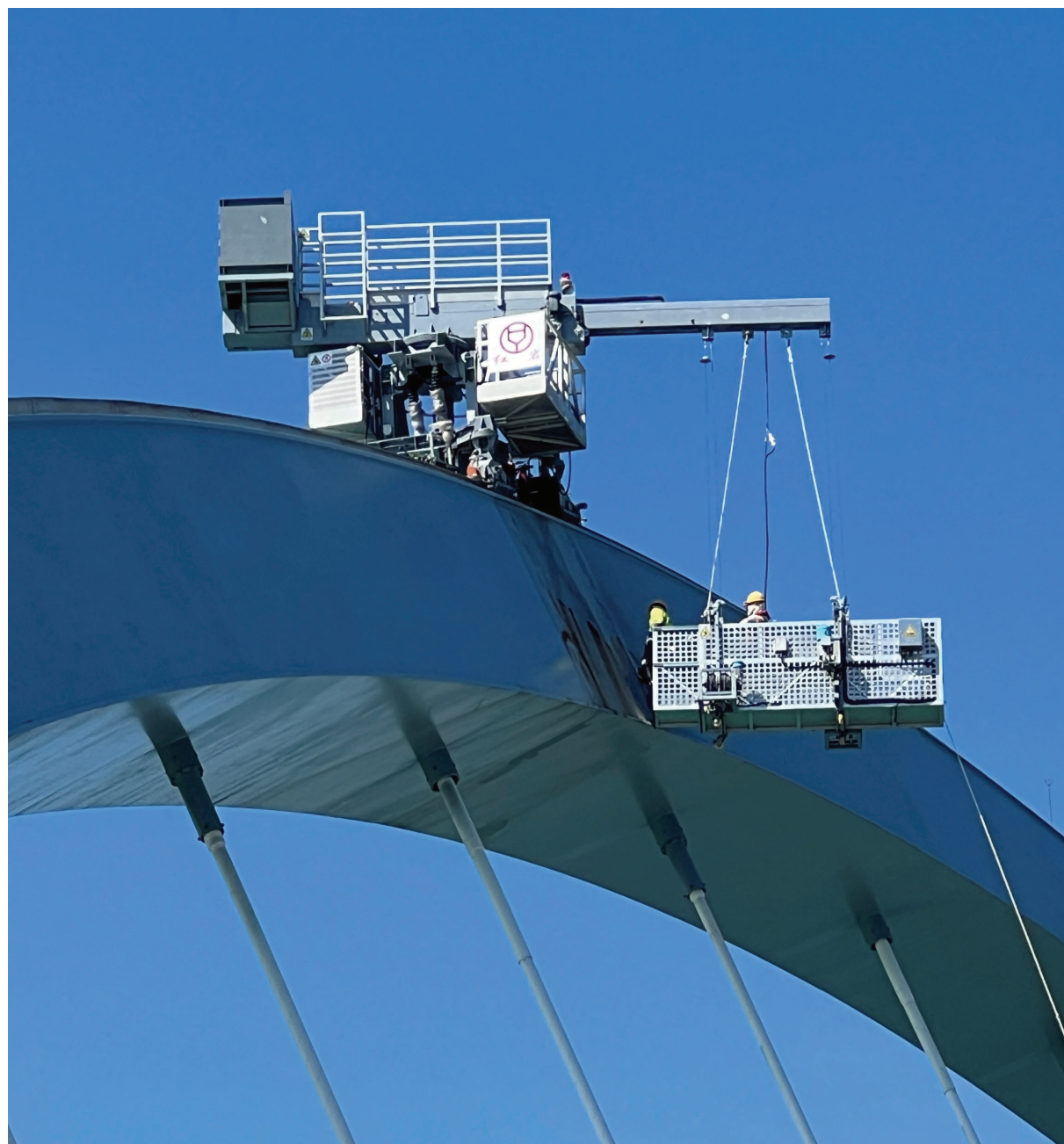
360度旋轉式機械吊臂及伸縮工作平台 360° mechanical arm and an extendable working platform
