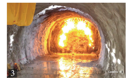
隧道爆破 Tunnel blasting
