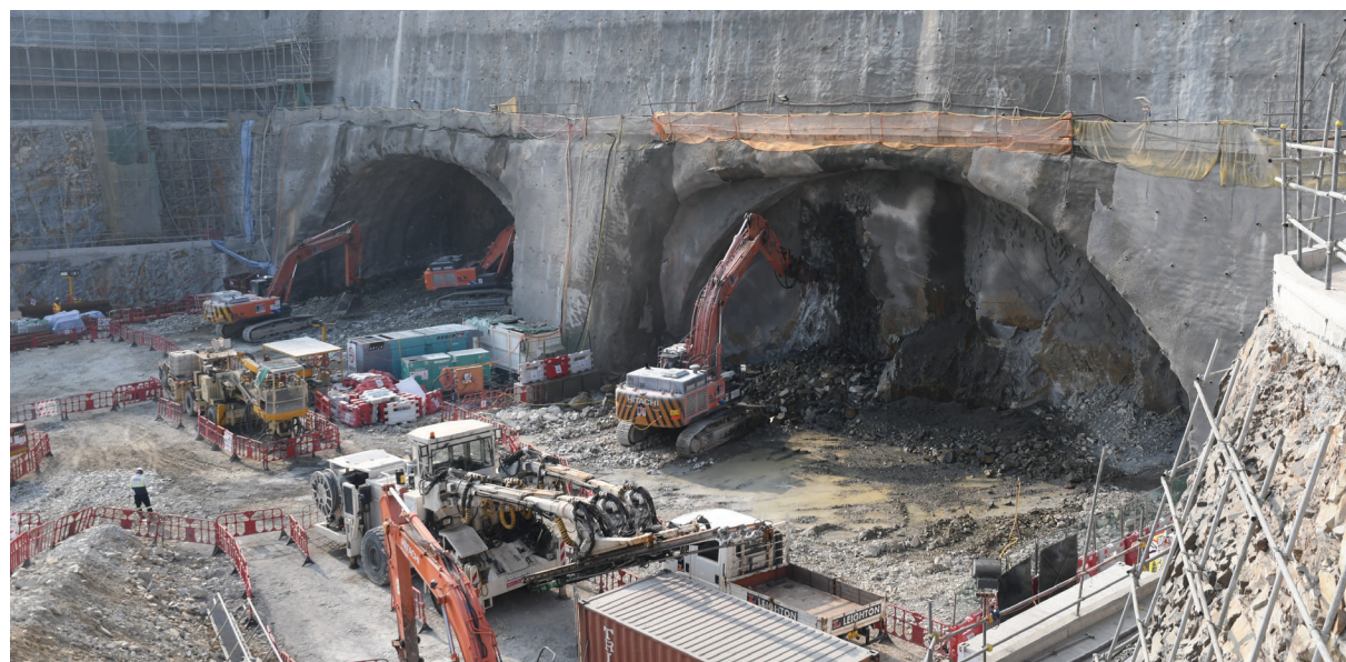
岩洞挖掘 Cavern excavation
