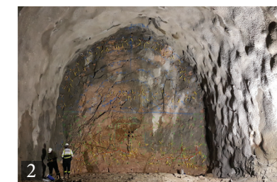
安裝爆炸品及接駁導爆索 Charging and hook-up
