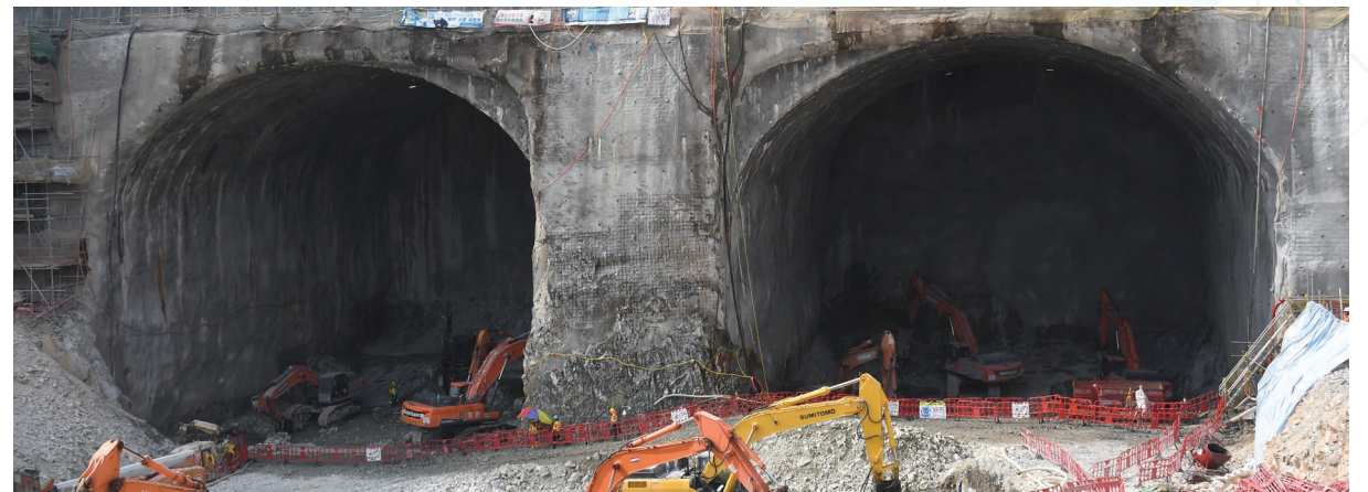
岩洞挖掘 Cavern excavation
