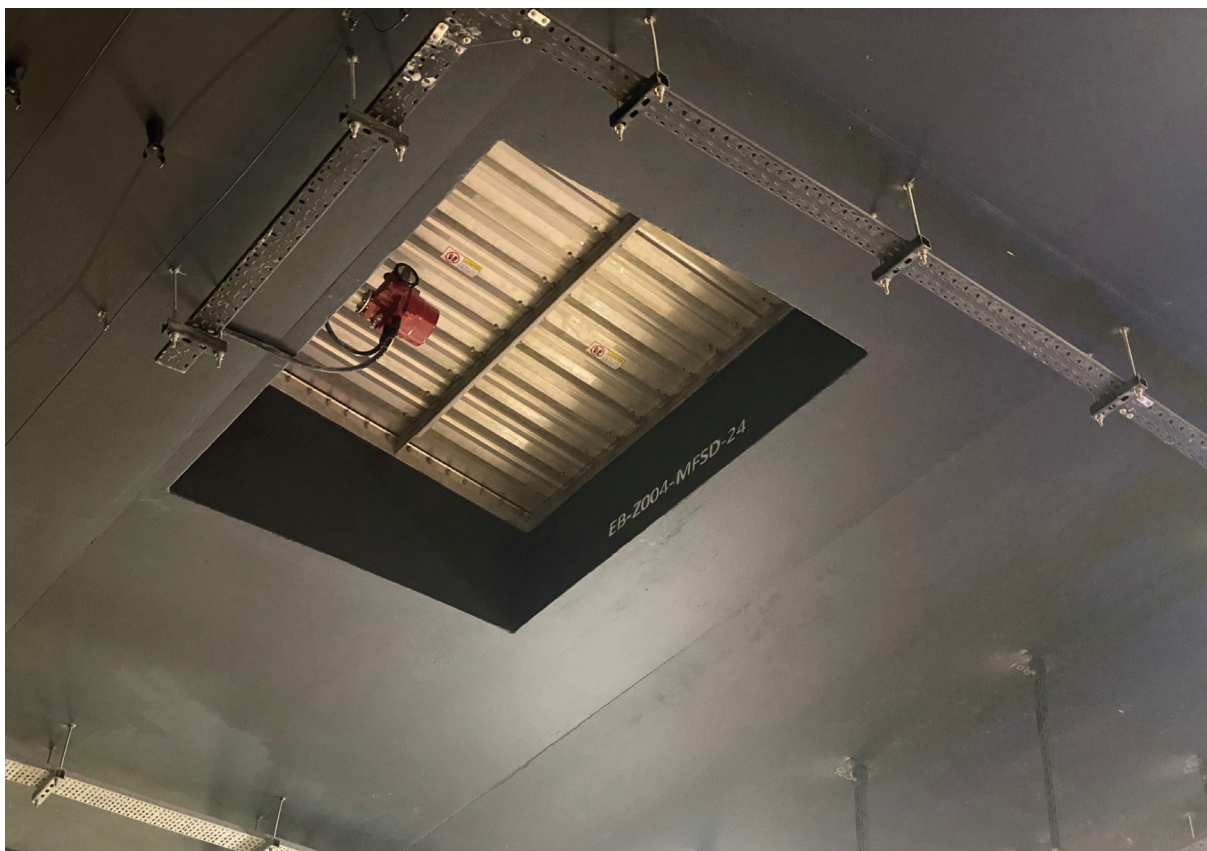
防火防煙風閘 Fire and smoke damper
